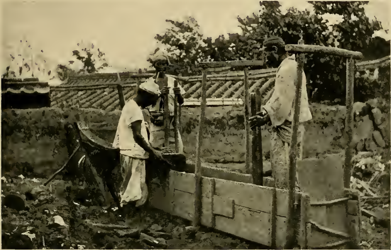
BRICK LAYING EXTRAORDINARY
